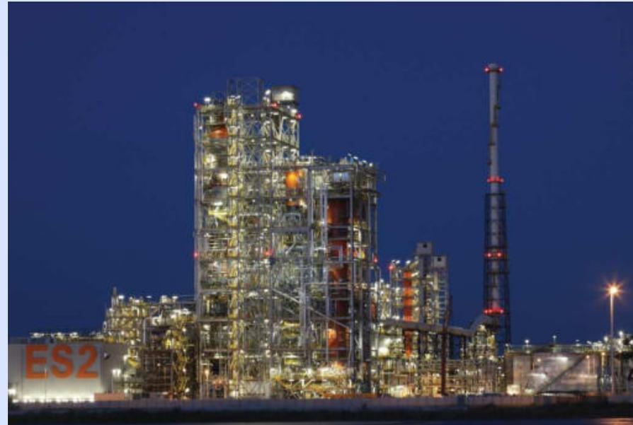
EST plant features n.2 x 2,000 t hydro-cracking reactors made of CrMoV + SS 347 Weld Overlay, supplied by GE-Nuovo Pignone, the largest ever built.
