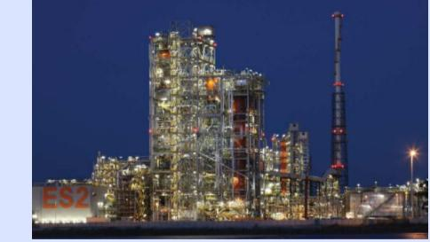
EST plant features n.2 x 2,000 t hydro-cracking reactors made of CrMoV + SS 347 Weld Overlay, supplied by GE-Nuovo Pignone, the largest ever built.
